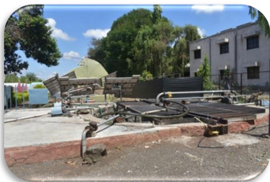
Water source- Open dug well
